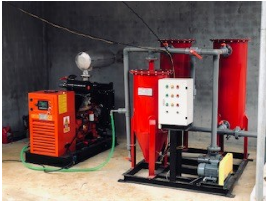
Figure 8. Model biogas generator system of the project deployed in Moc Chau - Son La.
